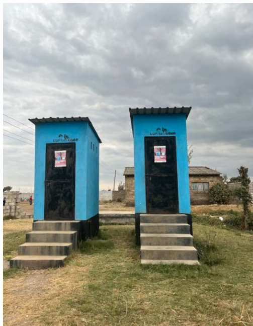
Figure 6: Safe pit latrines in Kanyama, constructed for residents through the partnership between Kanyama WT and the Bill and Melinda Gates Foundation
