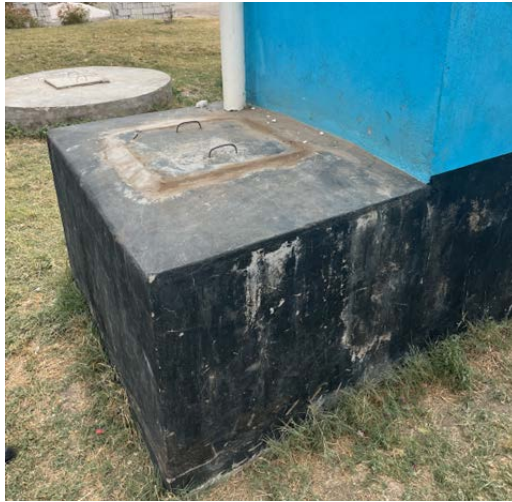
Figure 9: The lined pit of a safe pit latrine in Kanyama
